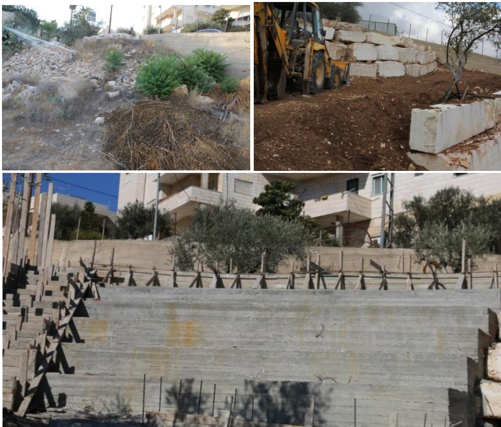
Area before and during infrastructure development. Bottom figure is concrete basis of educational Amphitheater.
