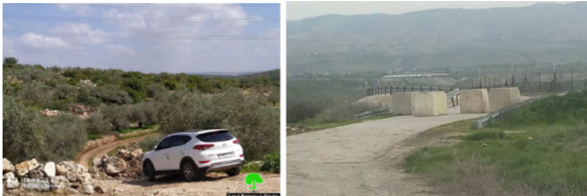
Figure 19 Examples of closures within the west bank via earth mounds or cement blocks (LRC 2021)
