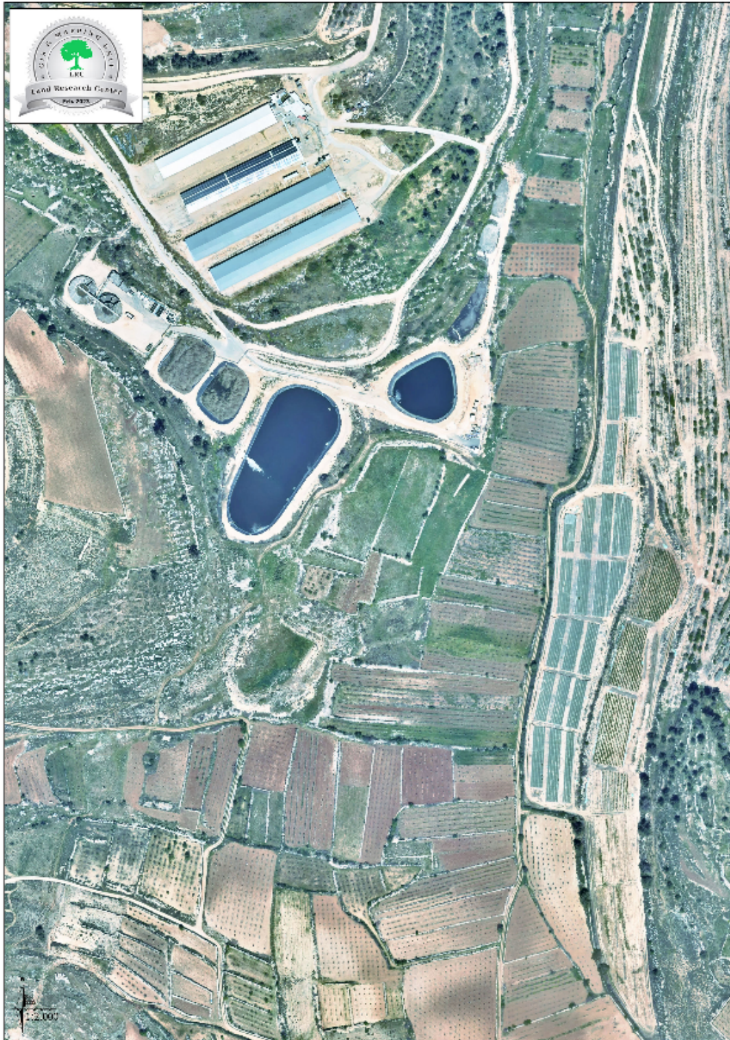
Fig. 4 Two images from LRC of Beit Ummar wastewater ponds, settlement, and Beit Ummar farmlands
