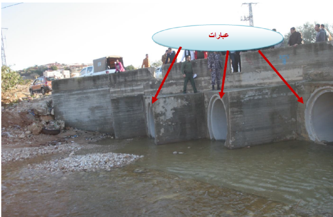
Figure 26 Wadi Beit Amin sewage from Shaar Hatikva mixed with rainwater.
