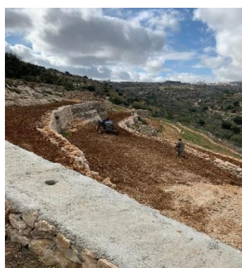
Photo 6.3: New terraces filled with new soil Photo 6.4: Use of mechanics on site mixtures on site Source: PCC, 2018
