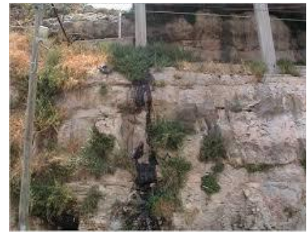
Photo 6.15: Leakage of wastewater from the cesspits in Battir locality
