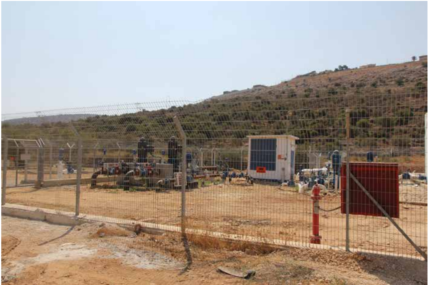
Figure 50. Water Station in Wadi Al Zarqa near Deir Ballout.
